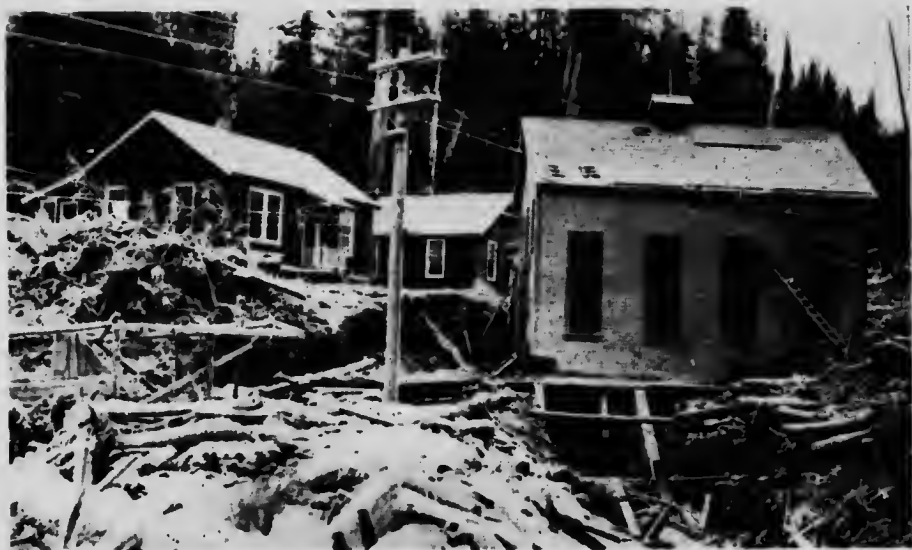
City of Prince Rupert-Woodworth Lake, near Prince Rupert. Front view of Power House.
